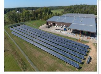
he second of ten 1.3-MW solar power plants for Hoosier Energy Power Network, a generation and transmission cooperative based in Bloomington, Indiana, is generating enough solar energy to power 150 homes in the region. The Cefox solar system uses 4,320 Canadian Solar modules on single-axis trackers, providing energy to UDWI and Daviess-Martin County REMC's customers. Cefox completed the turnkey EPC project with support from Recon in October 2015.
